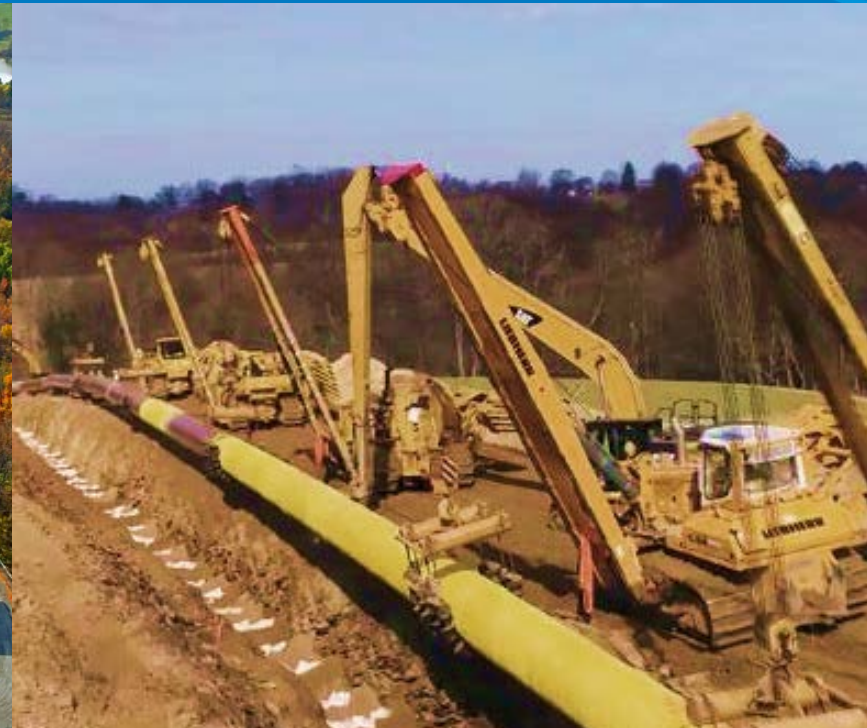
ATLANTIC SUNRISE CONSTRUCTION-TRANSCO PIPELINE Northeast Pennsylvania
