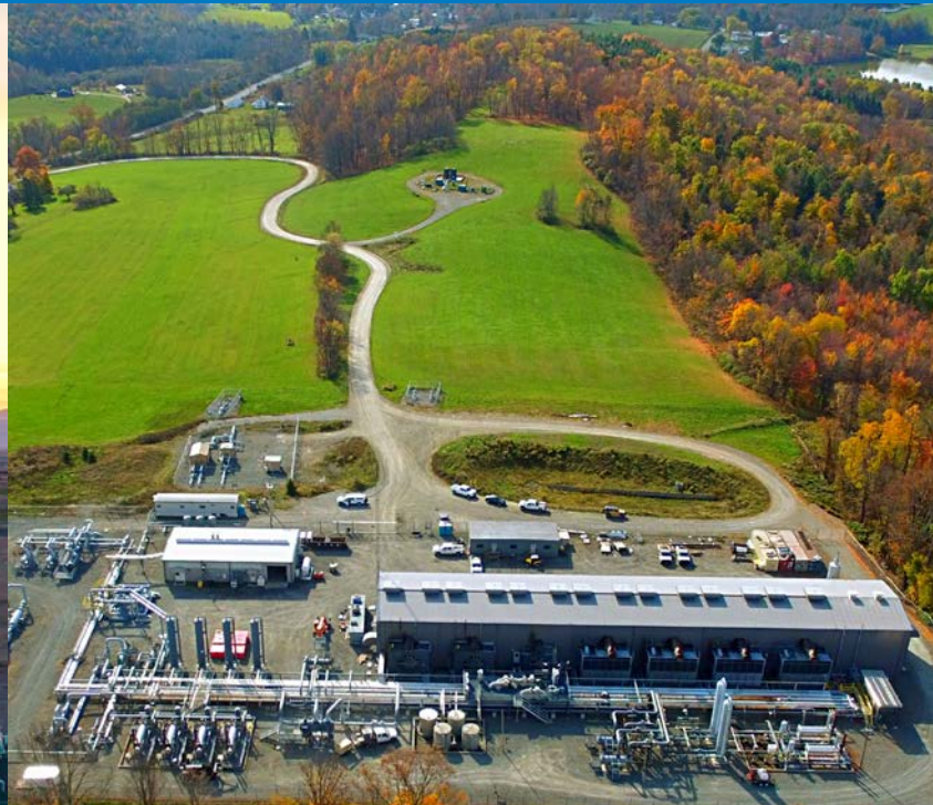
LATHROP COMPRESSOR STATION- SUSQUEHANNA Northeast Pennsylvania
