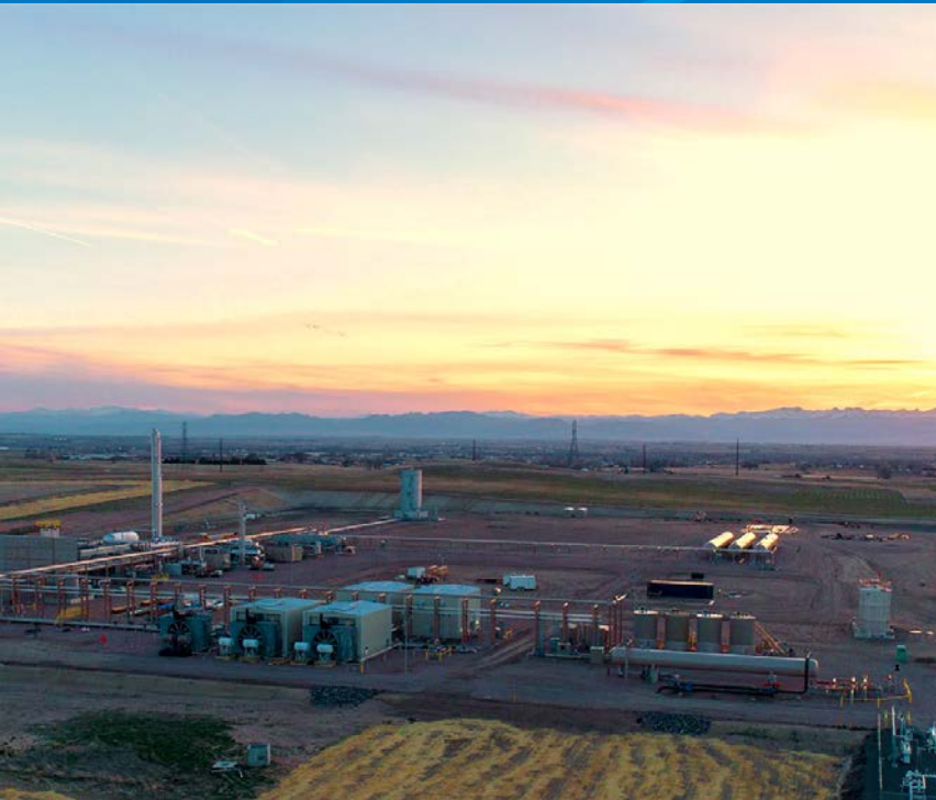
FT LUPTON PLANT- DENVER-JULESBURG DJ Basin, Colorado
