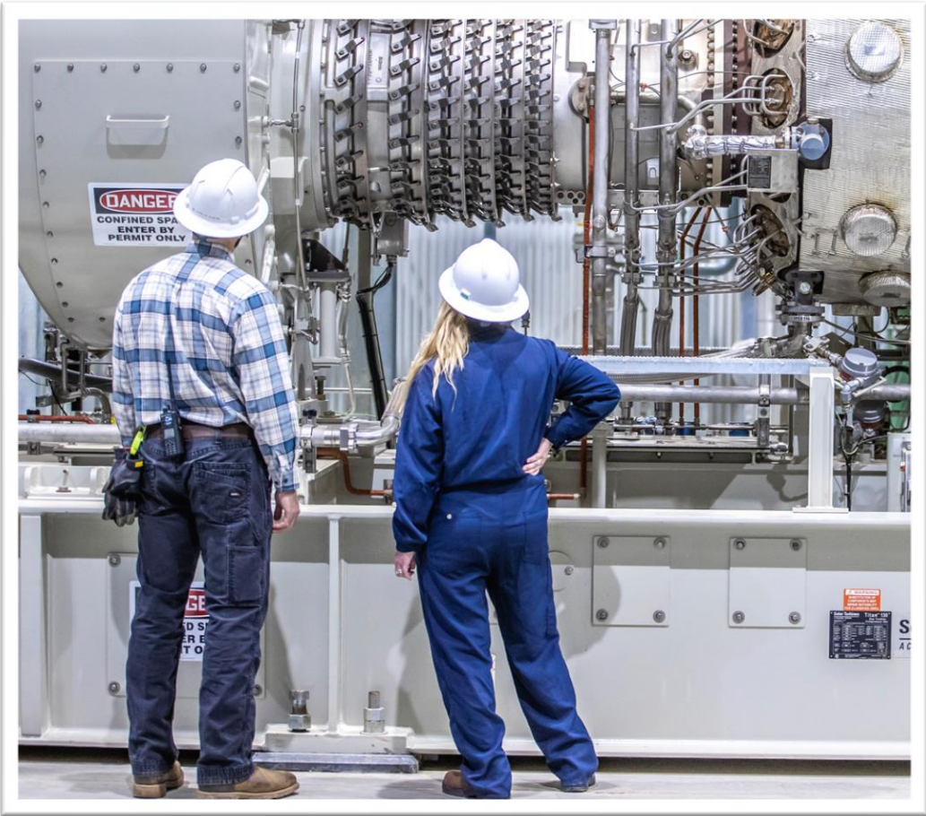
Transco Compressor Station 175 in Virginia
